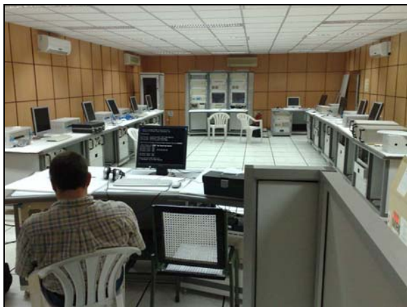
View of typical Strategic EW Station showing equipment cabinets and workstations
